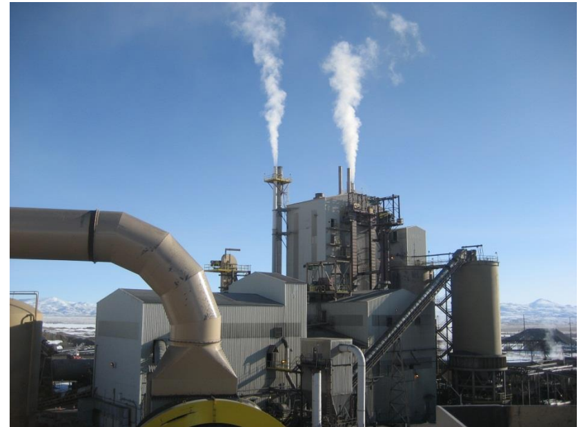
Jerritt Canyon Mine twin roasting facility, Elko Nevada.
