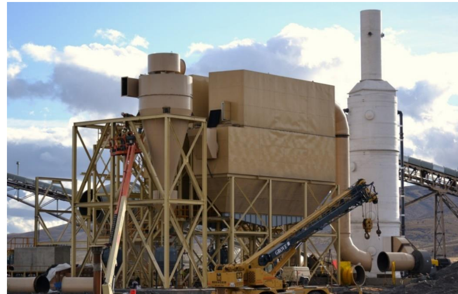
Constructing new ore dryer with mercury scrubbing stack, Jerritt Canyon Mine, Elko, Nevada
